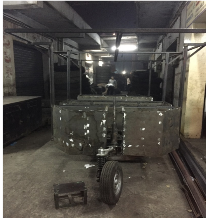
Fig. 5.6: Fabrication with Front covering
